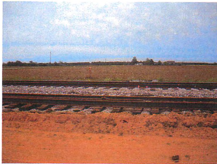
Existing railway, and pipeline monument
