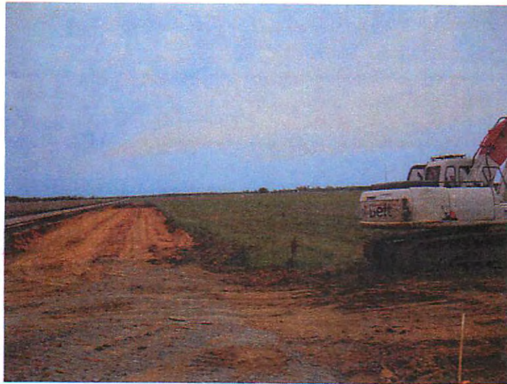
View Southeast Rail siding grading located on left
